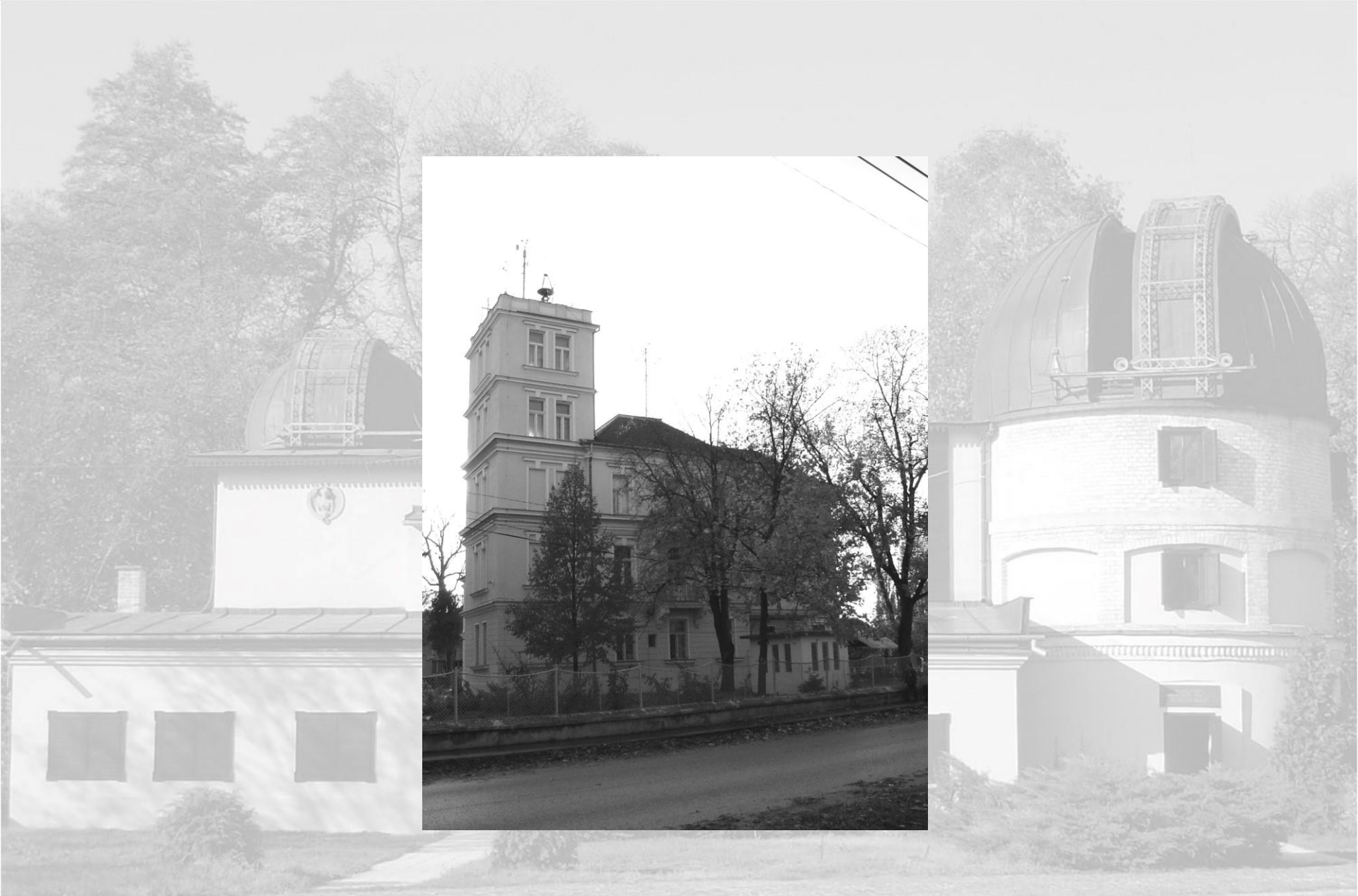
Building of geophysics and meteorological observatory in Hurbanovo
